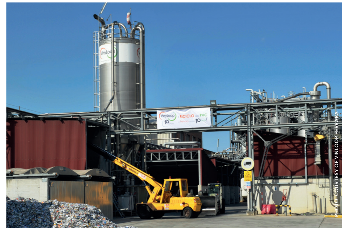
VinyLoop® (www.vinyloop.com) is a physical, solvent-based technology that can recycle difficult-to-treat, end-of-life PVC waste and produces high-quality R-PVC compounds.
